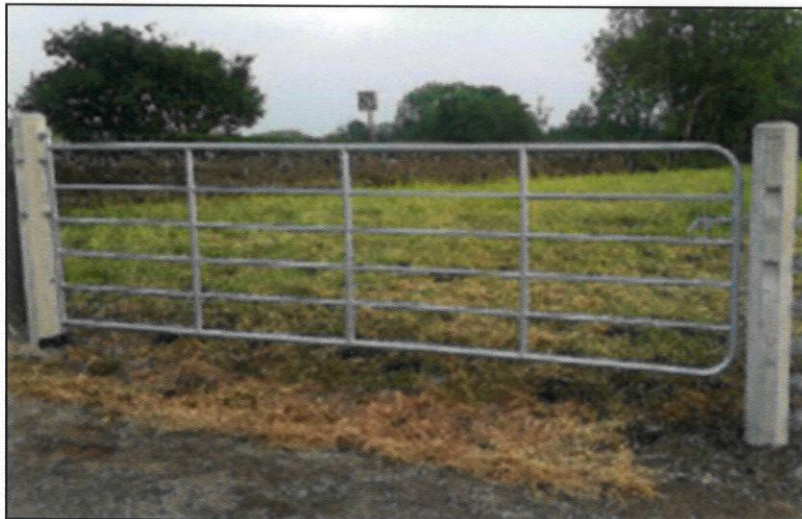
Typical 1.2m high Galvanised Steel Field Gate with Locking Mechanism
