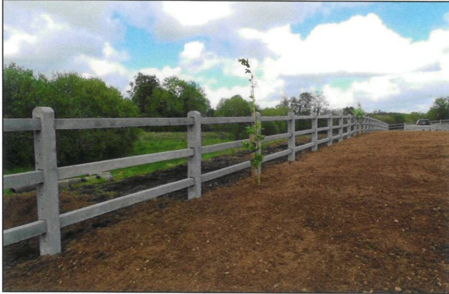
Typical 1.2m high 3-Rail Precast Concrete Fence
