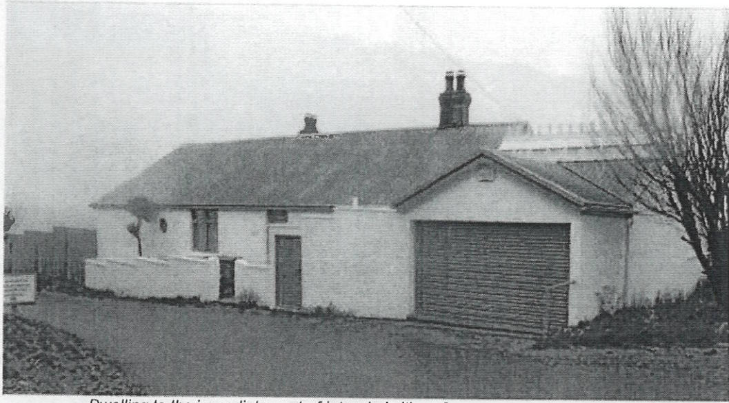
Dwelling to the immediate east of intended siting of concrete post and rail fence
